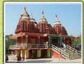
Sidheswar Temple Cement Nagar, Bargarh
