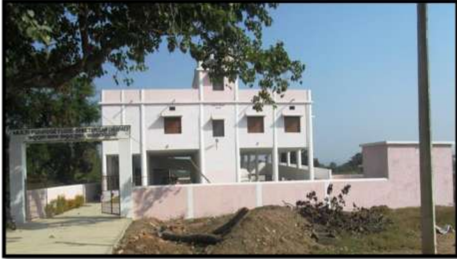
Multi-purpose Flood Shelter, Ganthiapali, Ambhabona Block
